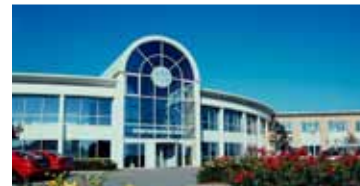
Pressalit Administration Testroom/Showroom Pressalitvej 1
