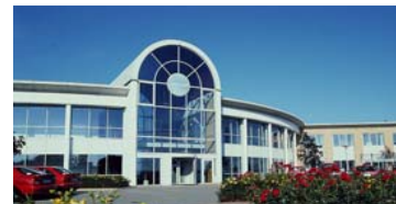
Pressalit Administration Testroom/Showroom Pressalitvej 1
